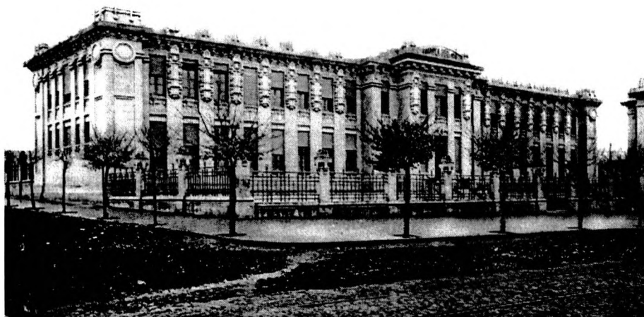
35. Fachada principal [anterior a 1935]
