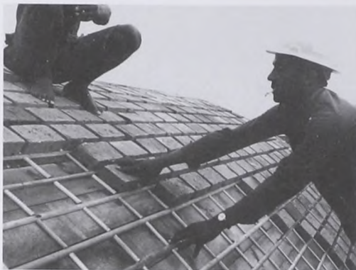
fig. 225: Small wood strips, nailed to the formwork to position the bricks. This stage is followed by the placement of reinforcing bars between the bricks and filling the joints with mortar.
