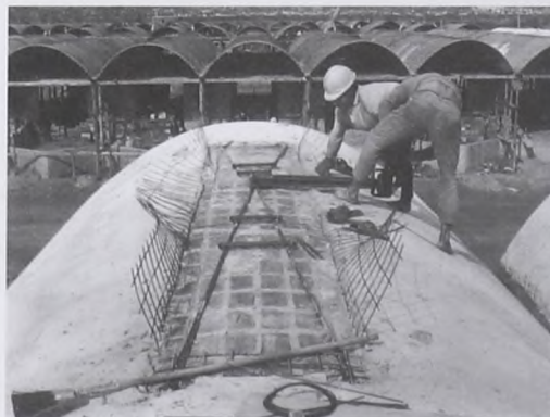
fig. 227: Pre-stressing the looped steel rods with a mechanical jack. The light steel welded mesh will be bent back and cemented to complete the roof.
