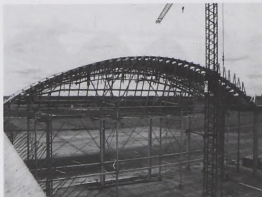
fig. 228: Metal framework and timber superstructure (ribs and plank-ing) of formwork for a vault of 98.5-foot (30-meter) span. Rails are placed just under the outermost steel pipe columns. During horizontal displacement of the form, the central columns do not play a structural role. (Lanas Trinidad wool warehouse, Durazno, ca. 1988)
