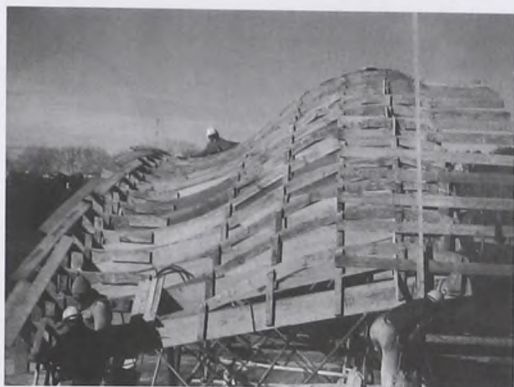
fig. 231: Timber ribs of the formwork, just before laying the surface planking
