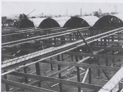
fig. 222: Small self-carrying vaults. In the foreground, the reinforced masonry "valleys" of what will be the laterally adjoining vaults can be seen; beyond, the wooden formwork for a series of barrel vaults.
