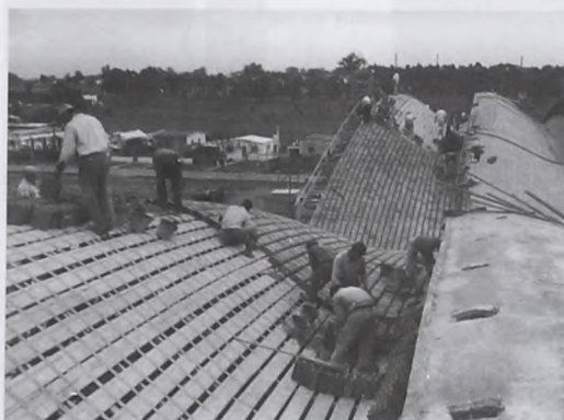
fig. 232: Discontinuous vaults with skylights. In the left foreground, wood strips on the planking control the location of the bricks. Reading into the center distance and back on the right side of the photograph, successive stages of the placement of brick, reinforcing, filling joints with mortar, and covering the bricks with a thin coating of cement are visible. The holes at the upper edge of the vault at the right allow the fixing of the vertical frames of the skylight. (TEM factory, Montevideo, 1960)
