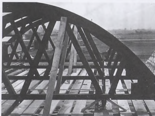
fig. 223: Timber trusses for the formwork in figure 222. The formwork moves on rails set on the timber platform.
